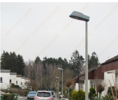
cobra head fixtures
