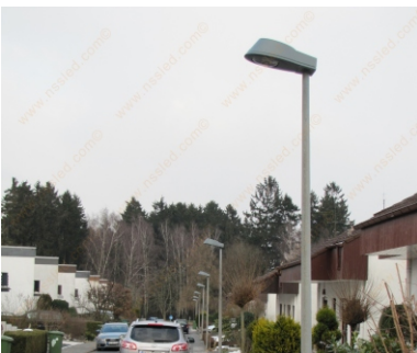
cobra head fixtures
